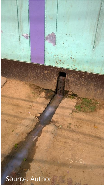
An open drain from a house.
