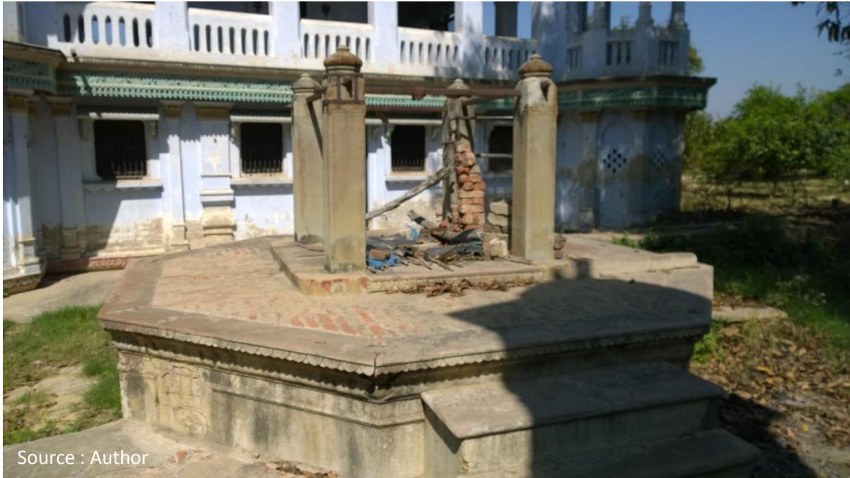
A well inside the premises of the structure.
