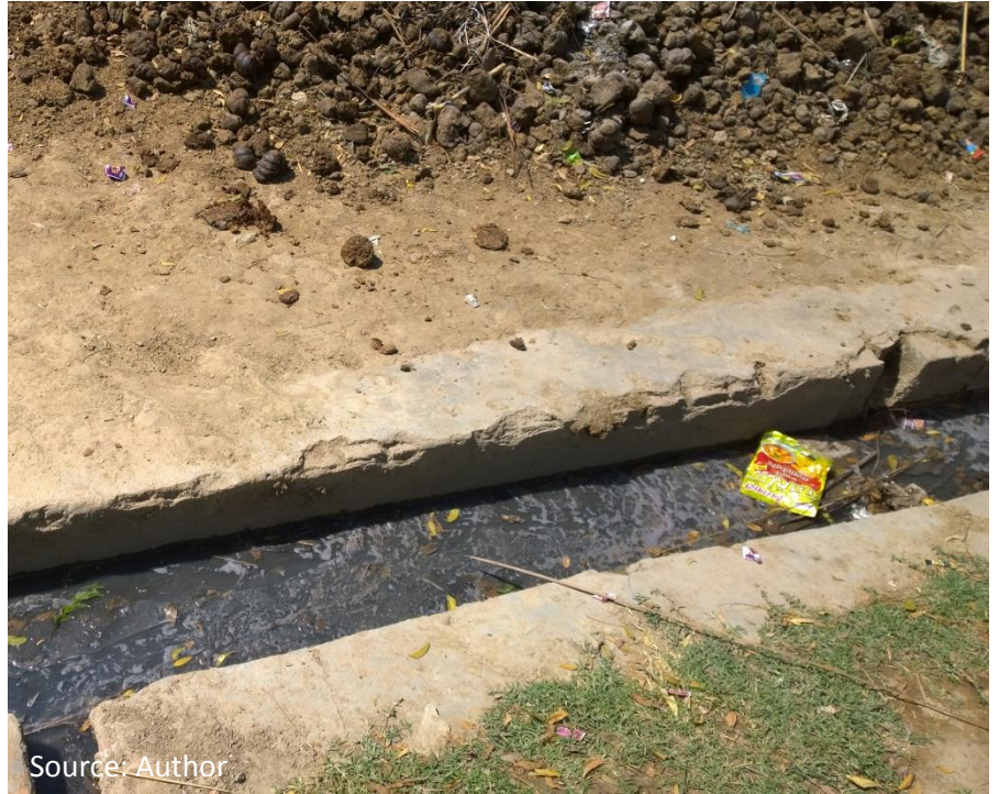
Stagnation of drains due to blockage by dumping of garbage in the drain.
