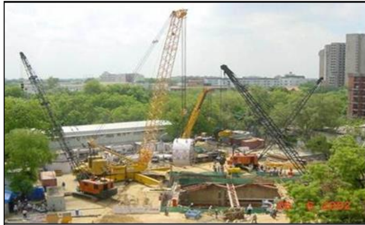
FIGURE 5.50: MAIN SHIELD ERECTION
