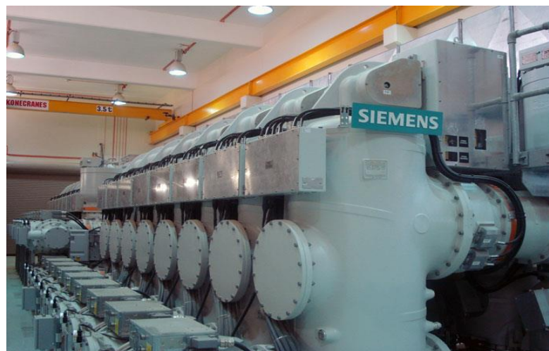
FIGURE 12.1 : GAS INSULATED SWITCHGEAR
