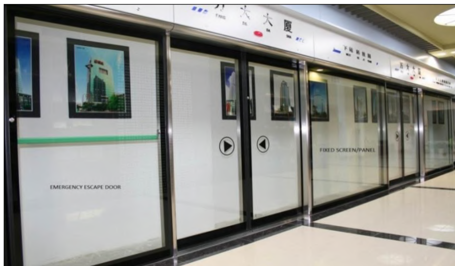
FIGURE 9.7: EMERGENCY ESCAPE DOORS & FIXED SCREENS/PANELS
