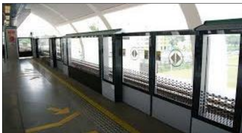
FIGURE 9.6: MANUAL SCREEN DOOR
