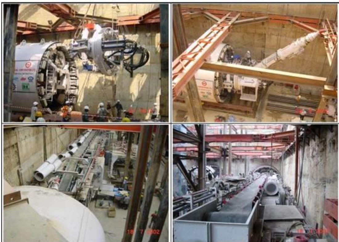
FIGURE 5.49: ERECTOR, SCREW CONVEYOR & BACKUP SYSTEM
