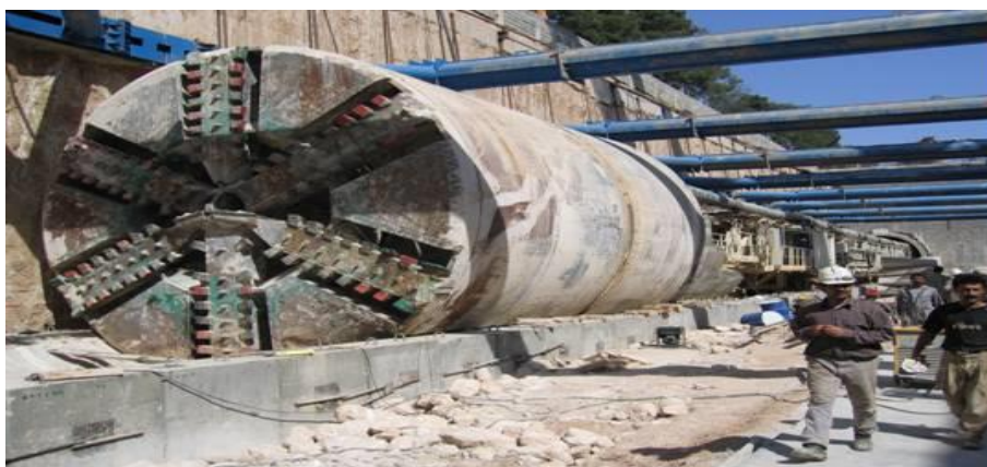
FIGURE 5.54: TBM PUSHED TO THE OTHER END OF THE STATION
