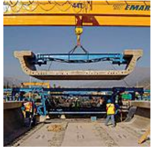
FIGURE 5.40: LAUNCHING OF U-CHANNEL GIRDER
