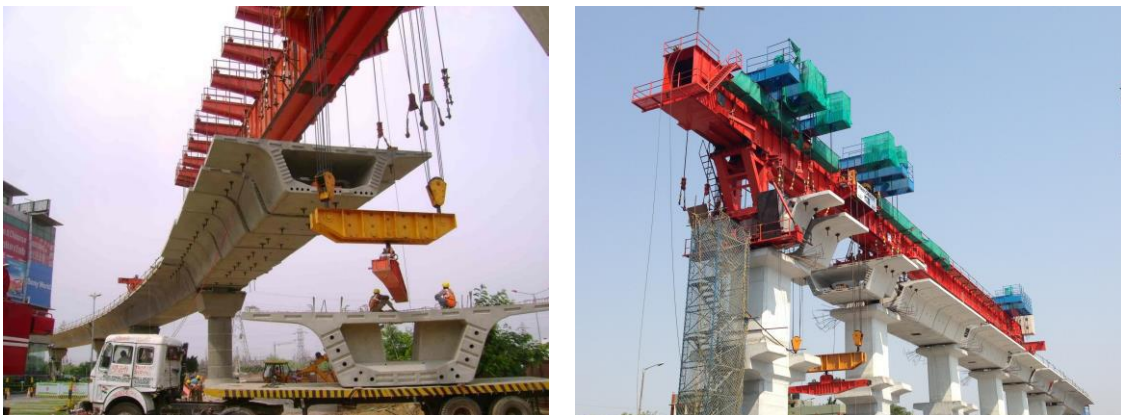
FIGURE 5.38: LAUNCHING OF BOX GIRDER SEGMENTS
