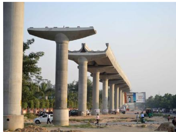
FIGURE 5.39: PRECAST U-CHANNEL SUPERSTRUCTURE
