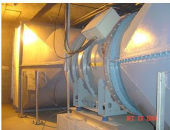
FIGURE 6.13: TUNNEL VENTILATION FAN & DAMPERS
