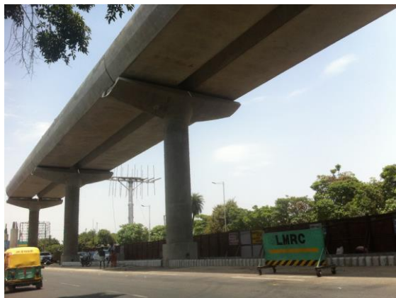
FIGURE 5.39: PRECAST U-CHANNEL SUPERSTRUCTURE
