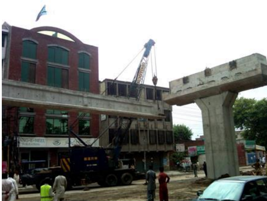
FIGURE 5.41: LAUNCHING OF I-GIRDER
