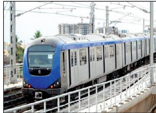
25 kV AC Overhead Catenary System
