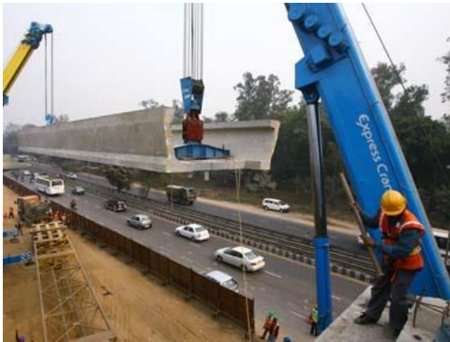
FIGURE 5.40: LAUNCHING OF U-CHANNEL GIRDER
