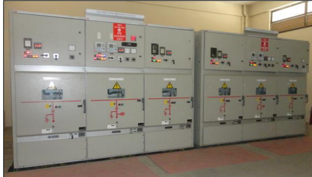
FIGURE 12.2: TYPICAL INDOOR AUXILIARY SUB-STATION (ASS)
