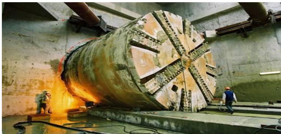
FIGURE 5.53: TBM THROUGH THE DIAPHRAGM WALL
