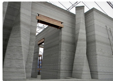
f) vertically printed, in-situ walls and columns: Total Kustom, USA
