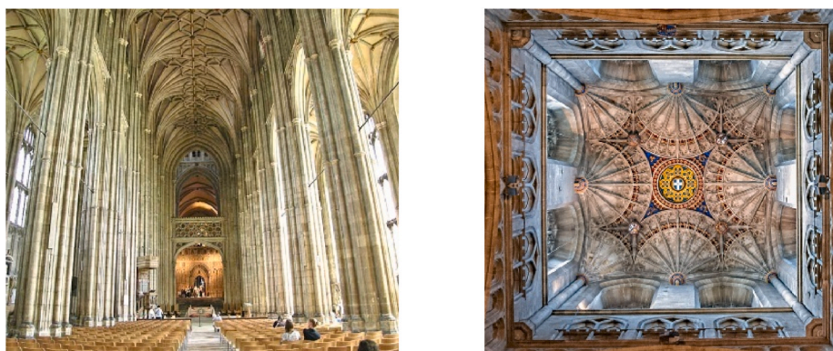
Fig. 8. Gothic vaulting: (a) main nave and (b) fan vault at the crossing, Canterbury cathedral, England.
