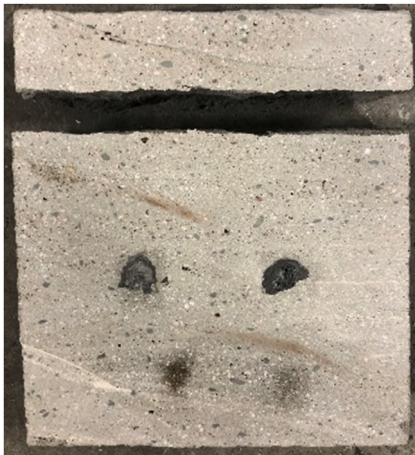
Fig. 27. C3DPC Sample 2 – Interlayer delamination.
