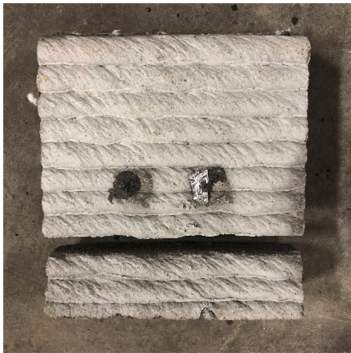
Fig. 21. 3DPC Sample 3 – Interlayer delamination.
