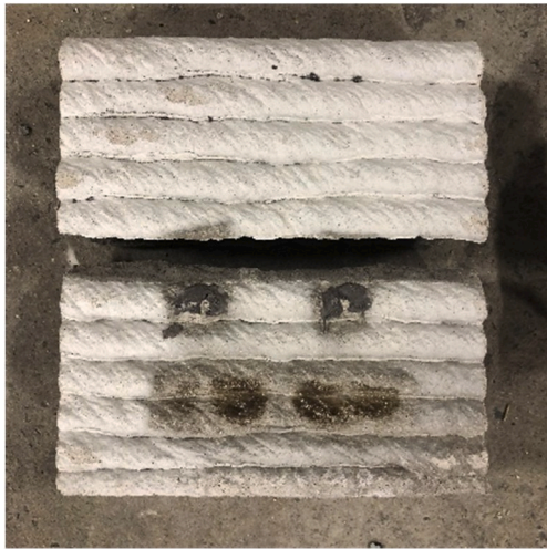
Fig. 20. 3DPC Sample 2 – Interlayer delamination.
