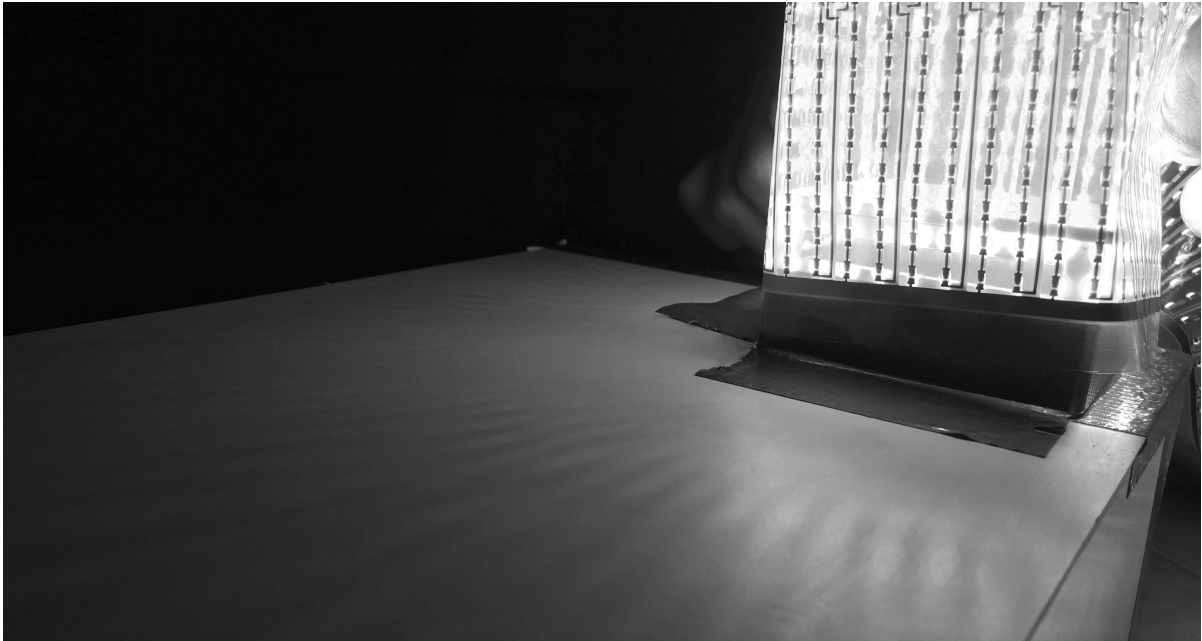
Fig Above: LED Film Used to produce diffused lighting. Product used : Cool Edge strip, 4000K Color Temp on a 1-10V dimmer.
